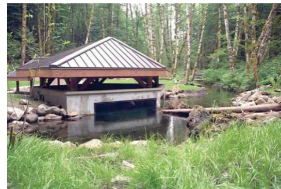
The developed facilities at Cascade Streamwatch include a unique underwater stream-viewing chamber along a restored side channel of the Salmon Wild and Scenic River. (BLM)
