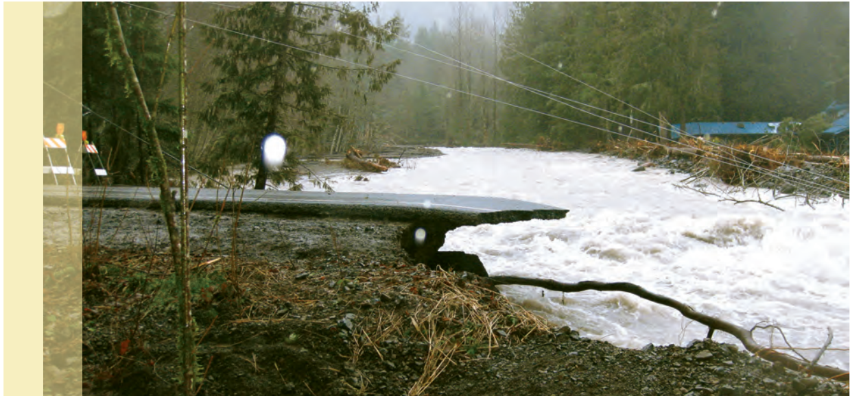
Washout of Lolo Pass Road by the Sandy River after rain and snow event, January 2011
