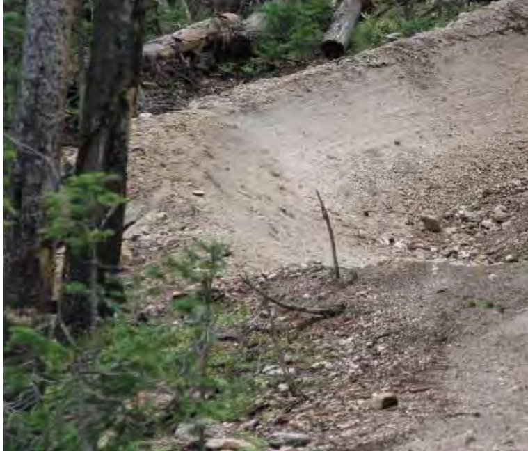
Constructed in-slope turns with sediment traps for run-off
