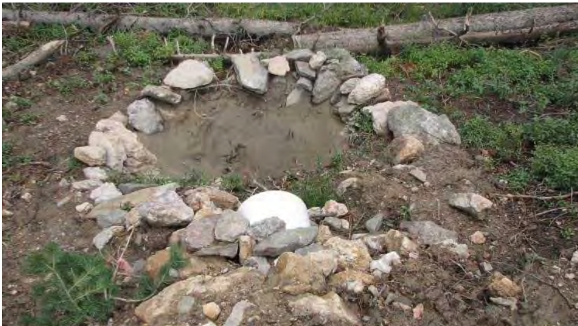
Rock fortify sediment trap at end of pipe and ensure depth of sediment trap is sufficient to remain underwhelmed during a minimum of 2 significant rain events
