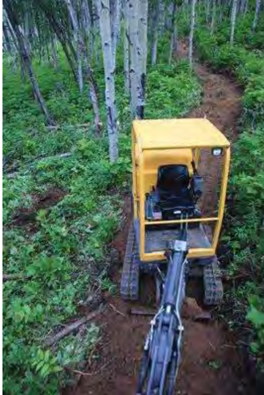
Above and Upper Right: Mini-excavator preparing narrow-excavated bike trail.
