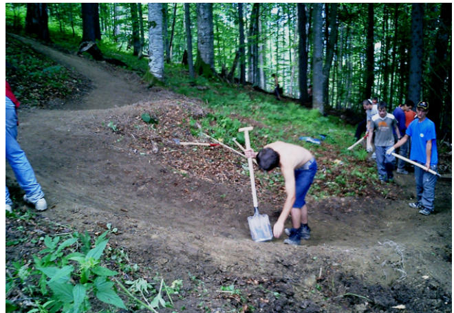
Lower Right - Hand Crew preparing final grade on narrow-excavated trail.
