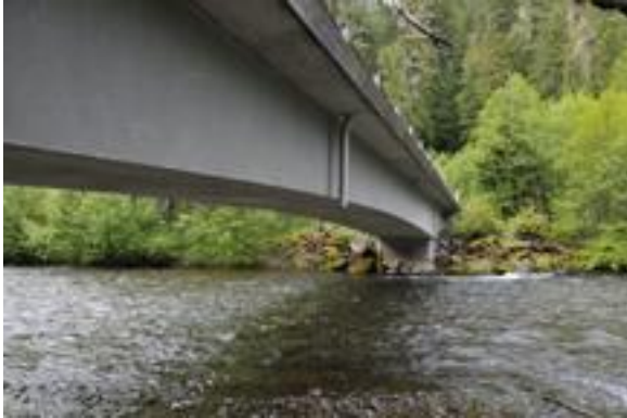
Photo of the 4650 bridge.
