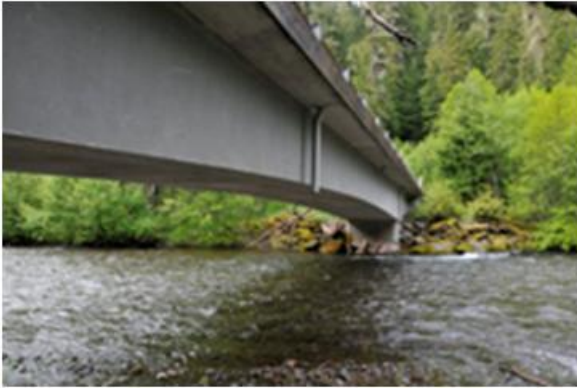
Photo of the 4650 bridge.
