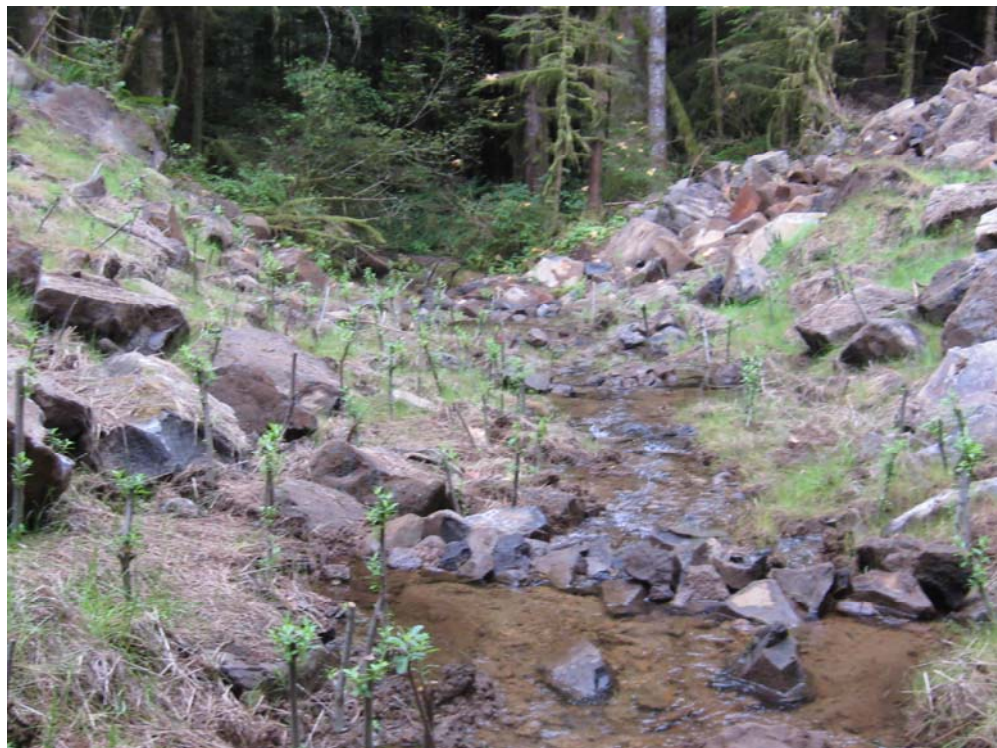
A Forest Service road once crossed this stream located on the Mt. Hood National Forest. The road was recently decommissioned restoring the stream to a natural condition and reducing the risk associated with the large fill located at this site.
