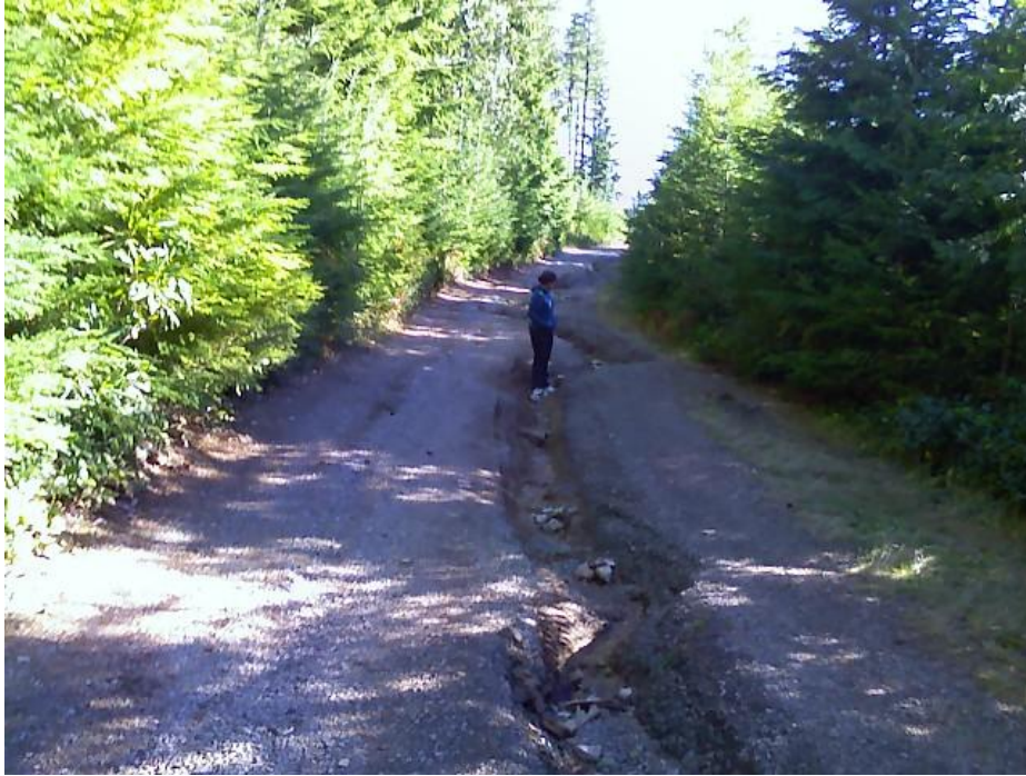
Figure 3.9. Example of gully erosion in the Wildcat Creek subwatershed.
